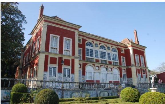
Figure 18 – The façade contours with a light colour.
