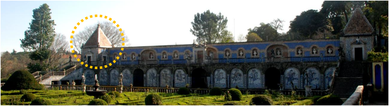
Figure 15 – The Kings Gallery and the Water Tank.
