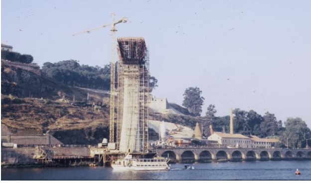
Figure 8. The construction phase (right bank - Oporto).
