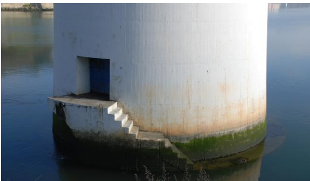
Figure 11. The pylon base after 20 years in use.
