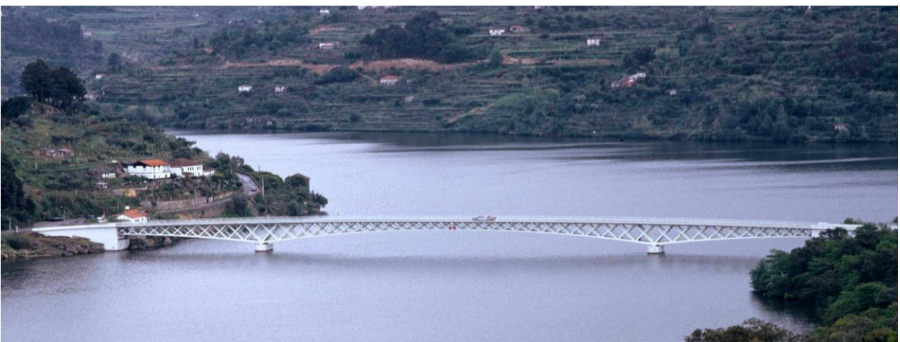
Figure 3. The 1973 Mosteirô roadway bridge by E. Cardoso.
