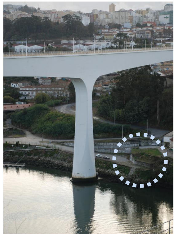
Figure 7. Trial painting tests area (left bank).
