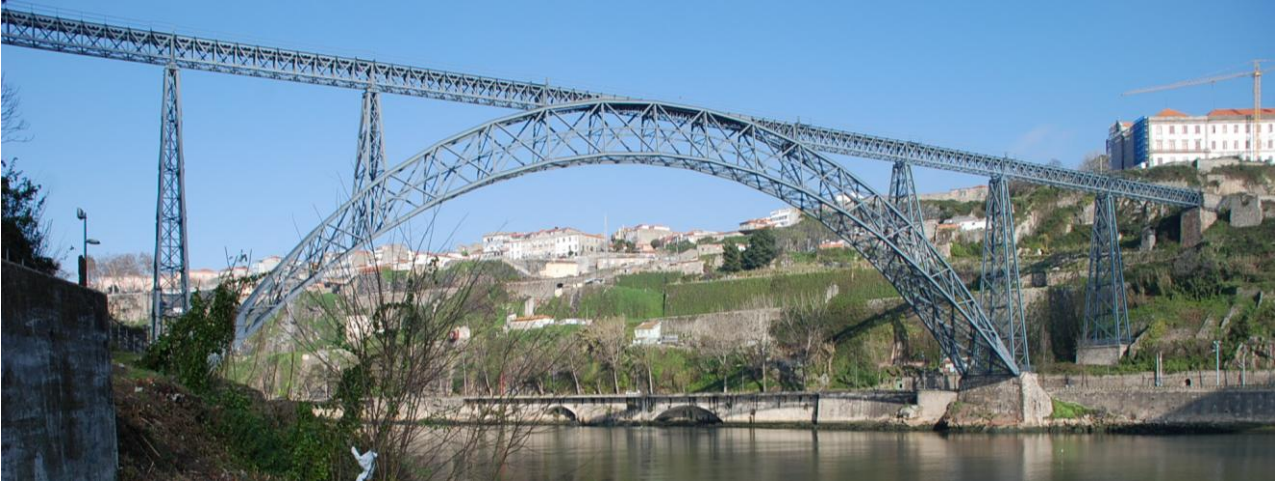
Figure 1. The 1877 Maria Pia railway bridge by G. Eiffel.
