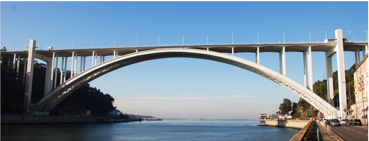
Figure 2. The 1963 Arrabida highway bridge by E. Cardoso.
