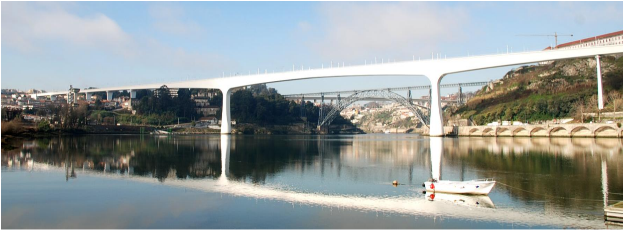
Figure 4. The 1991 São João railway bridge by E. Cardoso.
